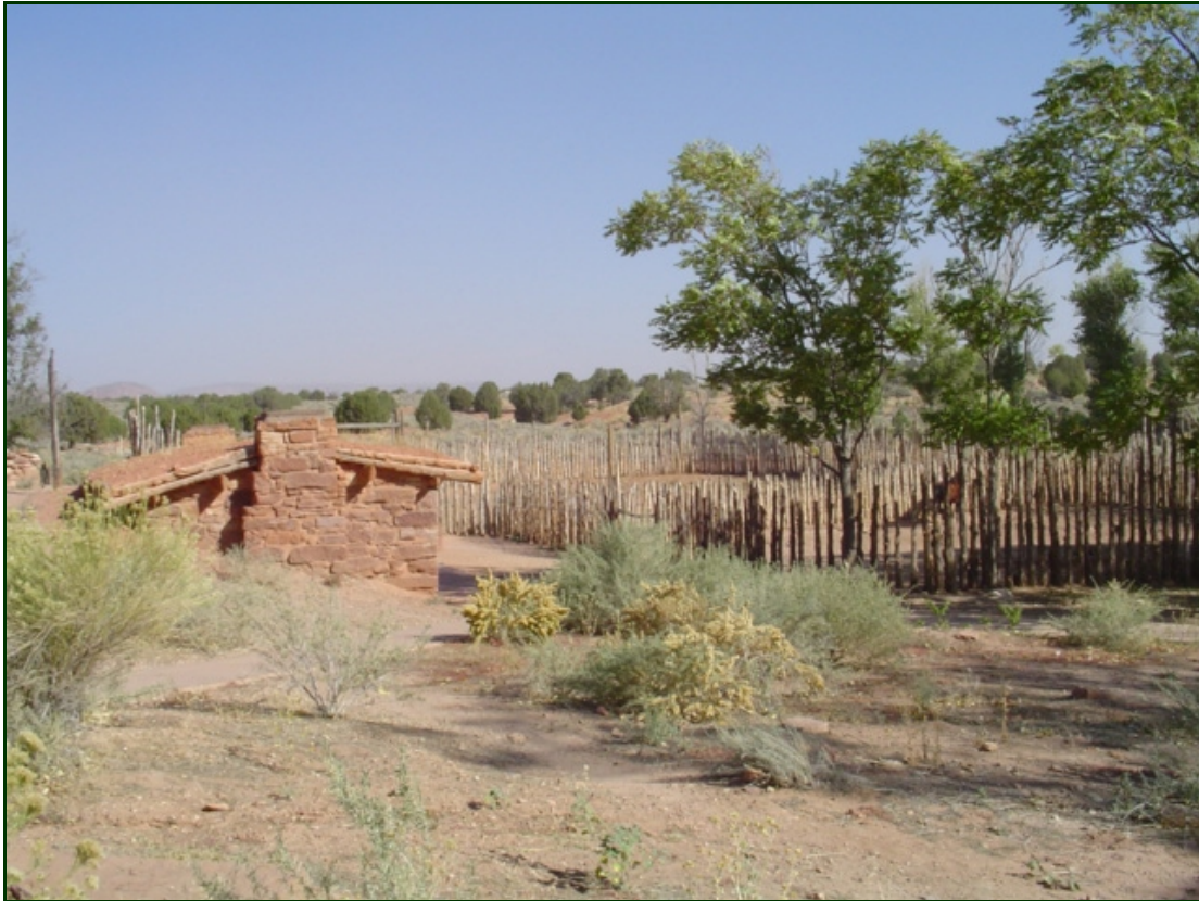
Dugout at Pipe Springs National Monument. Photo by author.
